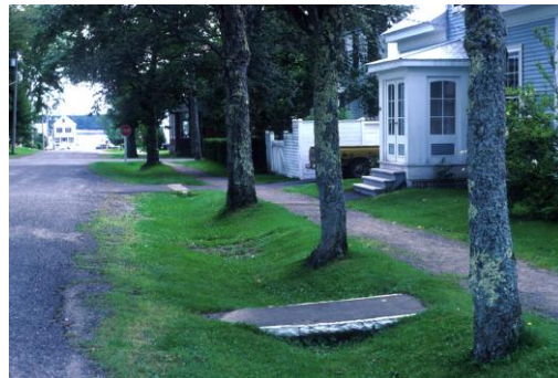
Fig. 11 Swales can easily serve in place of curbs, even when density is more than two or three dwellings per acre.
