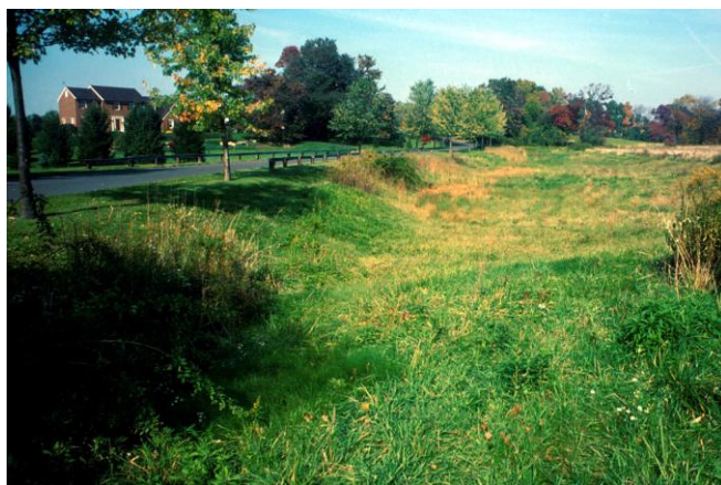
Fig. 11 Swales can easily serve in place of curbs, even when density is more than two or three dwellings per acre.
