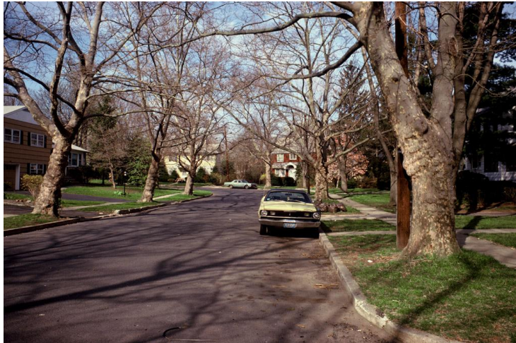
Fig. 19 This curve, along which my childhood home sits, in Cranford NJ, measures only 72 feet in radius. Such radii are far more effective than any speed sign or bump in terms of calming traffic moving through the neighborhood.
